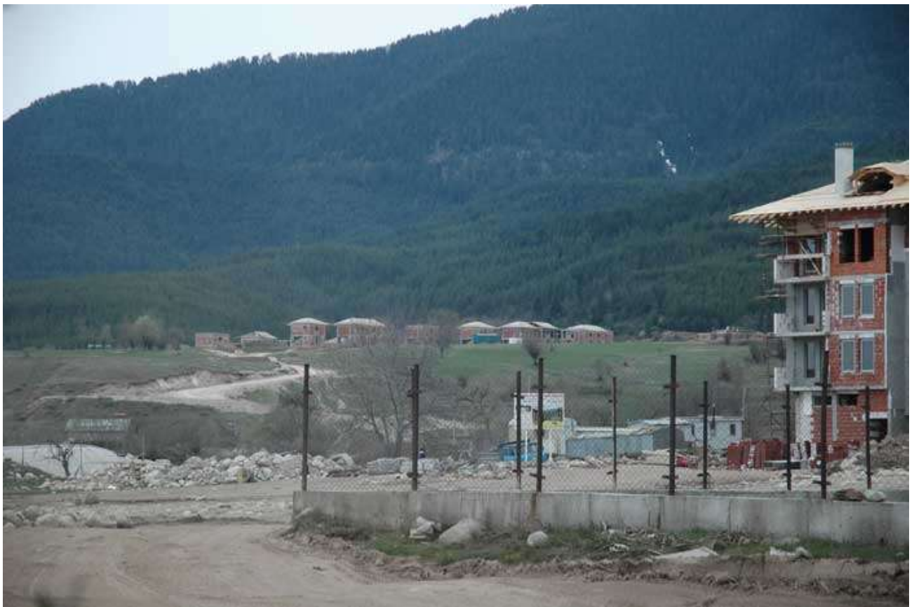
13. Buildings in Bansko
