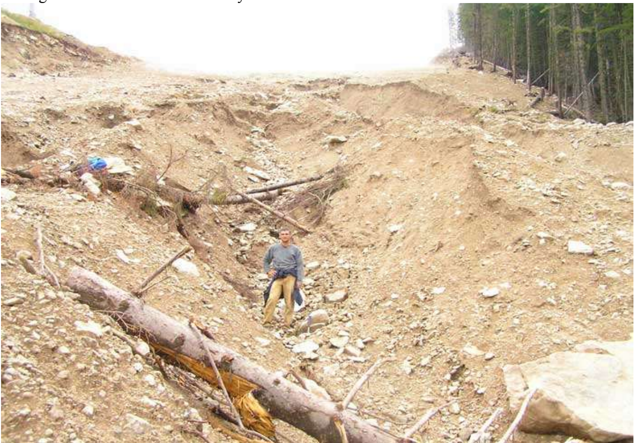
4. The consequences of excavation works
