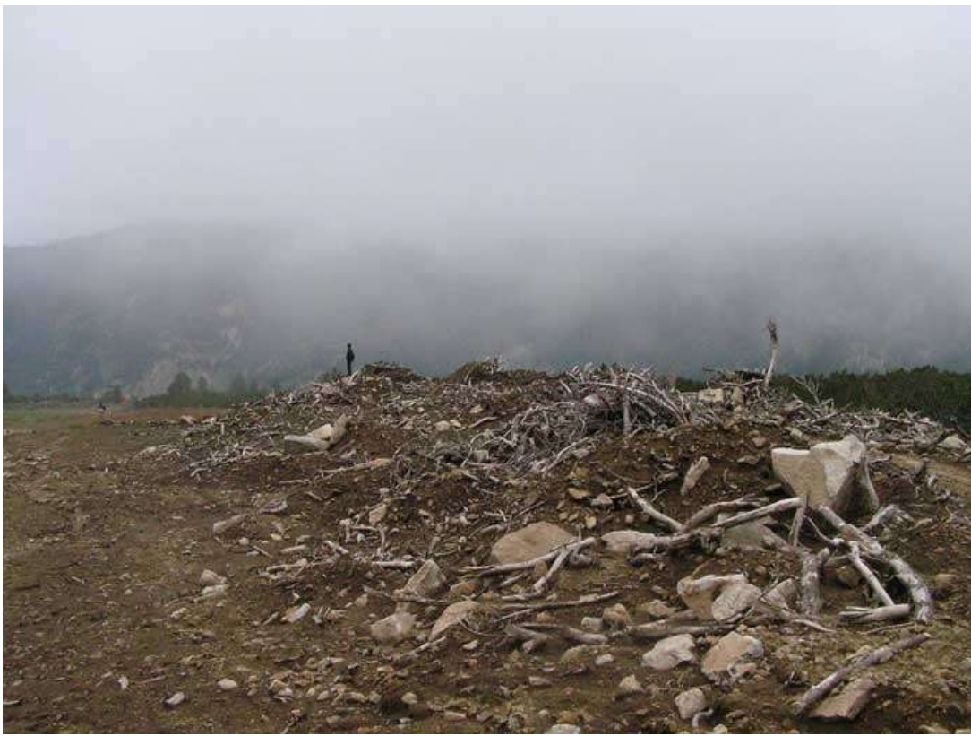
23. Fill work for the construction of the ski slope
