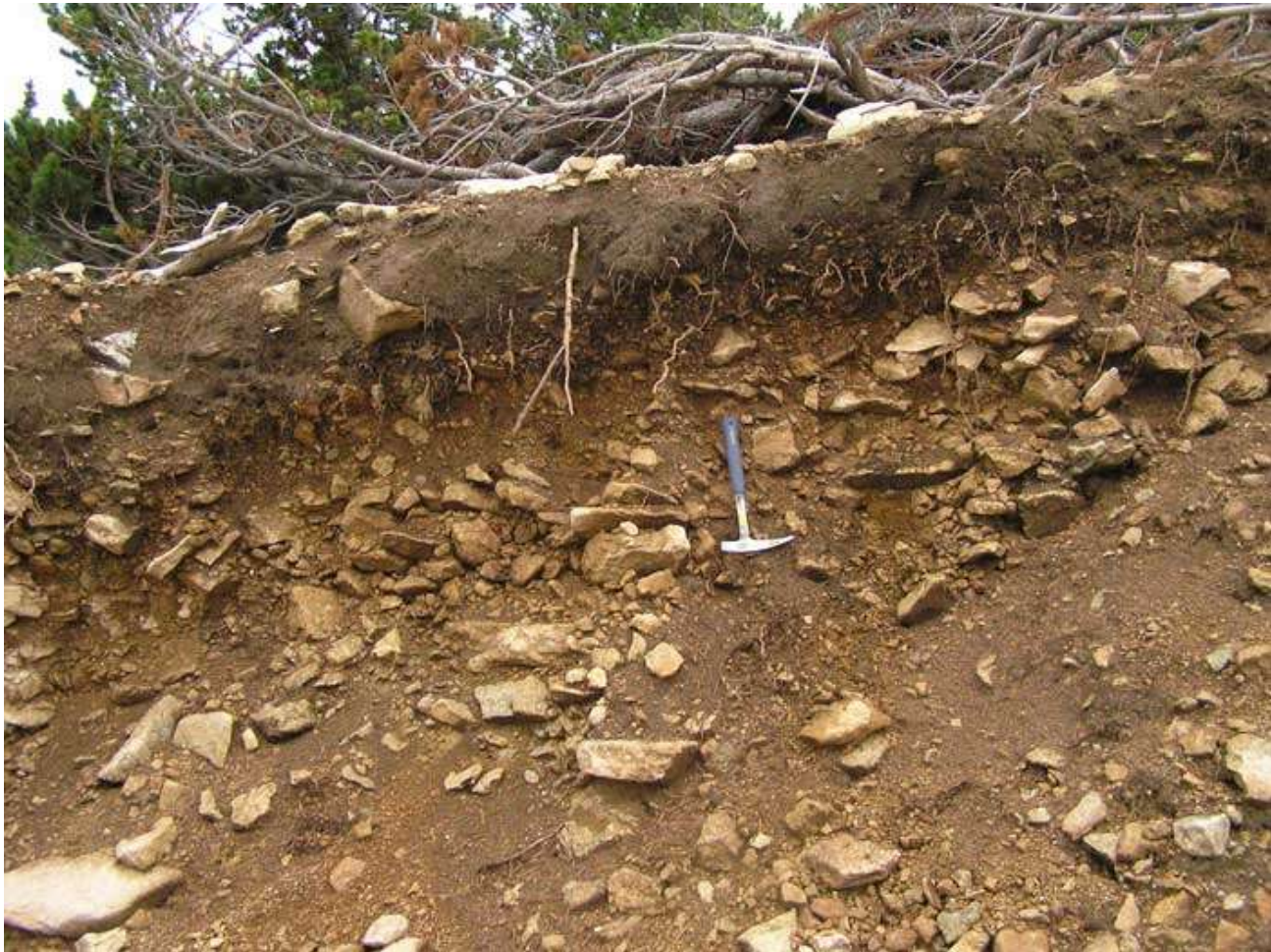
22. Fill work for the construction of the ski slope
