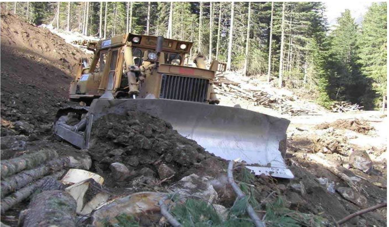
4. The consequences of excavation works
