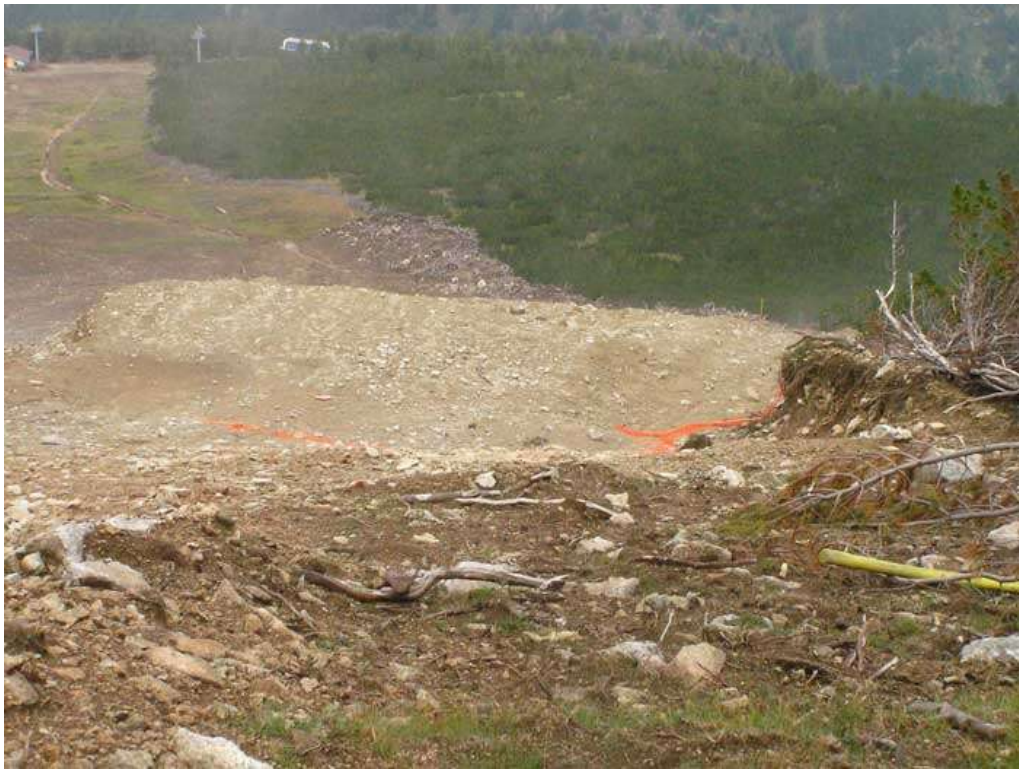
21. Fill work for the construction of the ski slope
