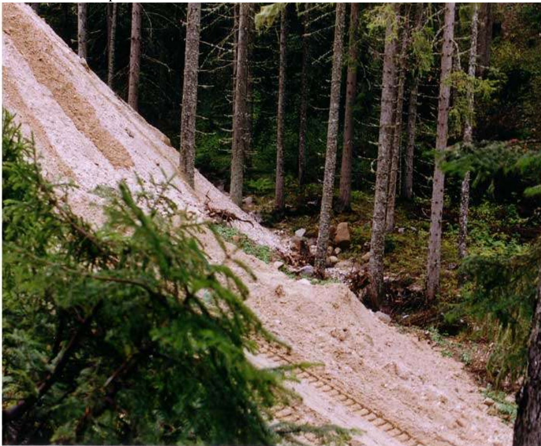
5. Construction and earth piling on the river beds
